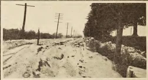
WAR-TIME DESTRUCTION OF OHIO ROADS. TOP—TAR MACADAM ROAD NEAR SANDUSKY, BROKEN DOWN BY HEAVY TRUCKING OVER A WEAK FOUNDATION. BOTTOM—BRICK ROAD IN SUMMIT COUNTY, DESTROYED BY HEAVY TRUCKS AND REPAIRED WITH 8-INCH CONCRETE FOUNDATION, MONOLITHIC TYPE.
